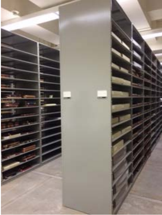
Example: Covered rails for future mobile shelving and example of horizontal volume storage with extra shelves
